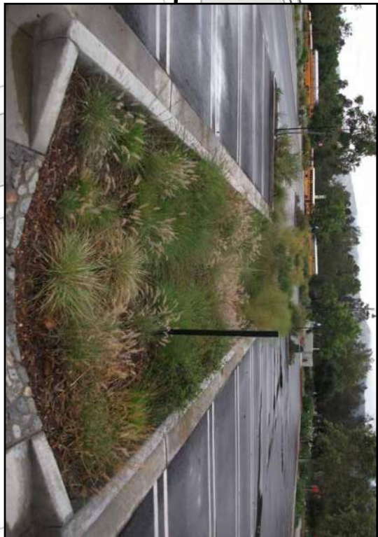
Parking Lot with Stormwater Basins
