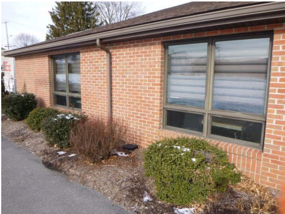
Photo #2 – No damage to exterior wall finishes noted
