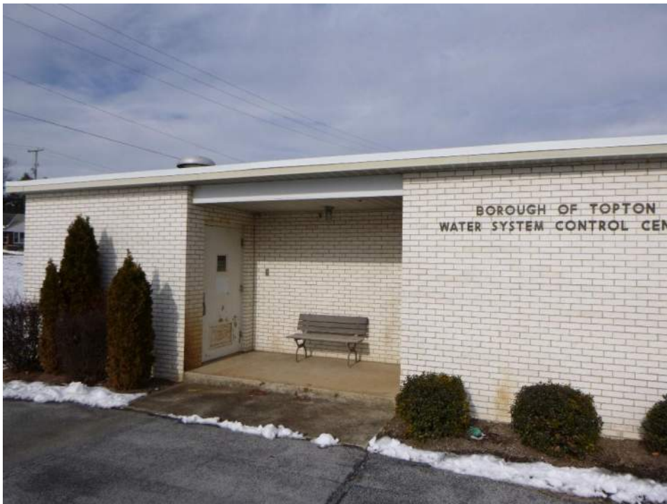
Photo #10 – No cracking or movement of Water Control building
