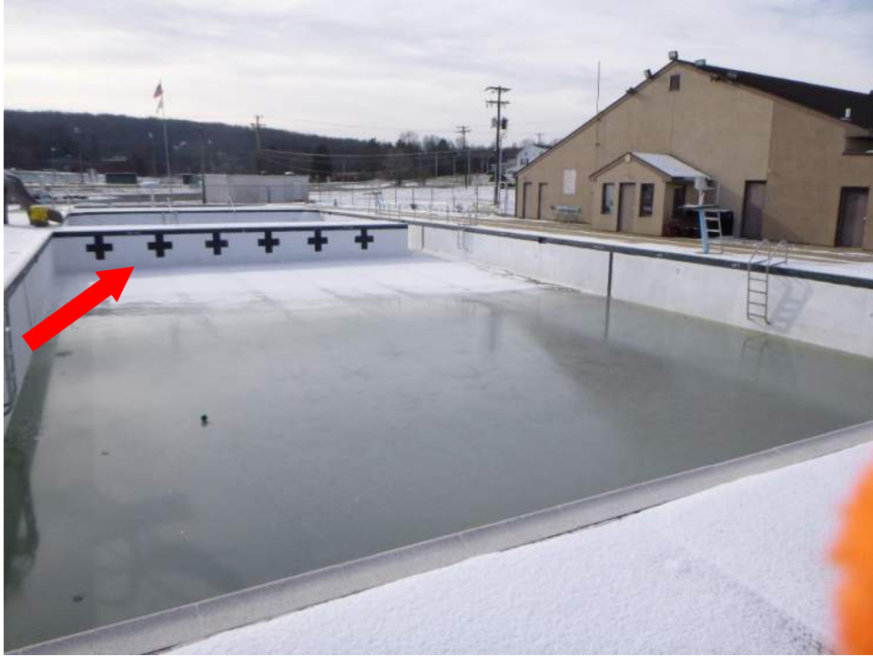
Photo #5 – Larger pool, and dividing wall (arrow)
