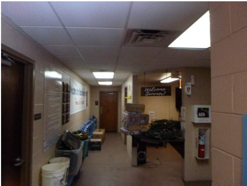
Photo #4 – No cracking or movement of slab or wall finishes
