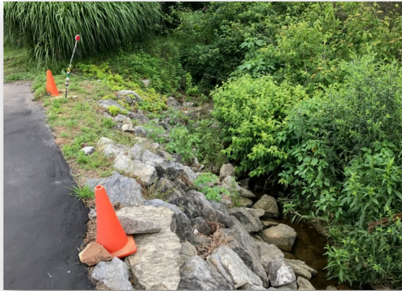
Photo 14: View of Tributary where steep embankment has been reinforced with rip rap
