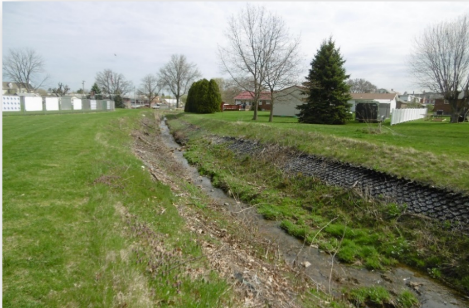
Photo 2: View looking North of Toad Creek. Bank stabilization using geogrid not successful
