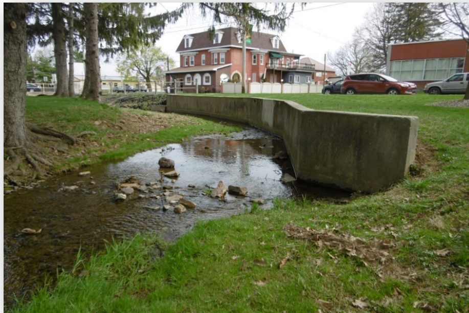
Photo 4: East side of Toad Creek reinforced with concrete wall, near E Barkley Street
