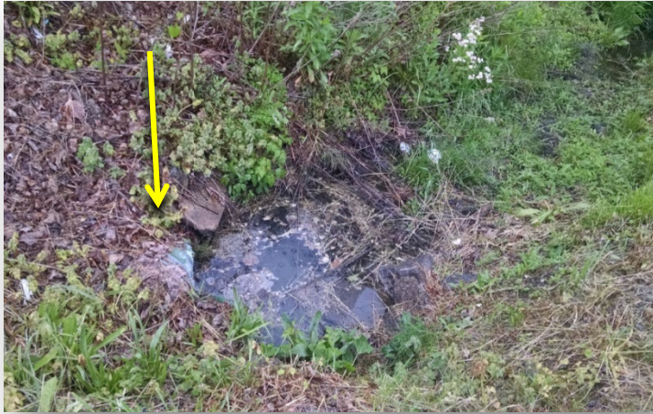
Photo 7 (Above): Corrugated metal pipe partially submerged
